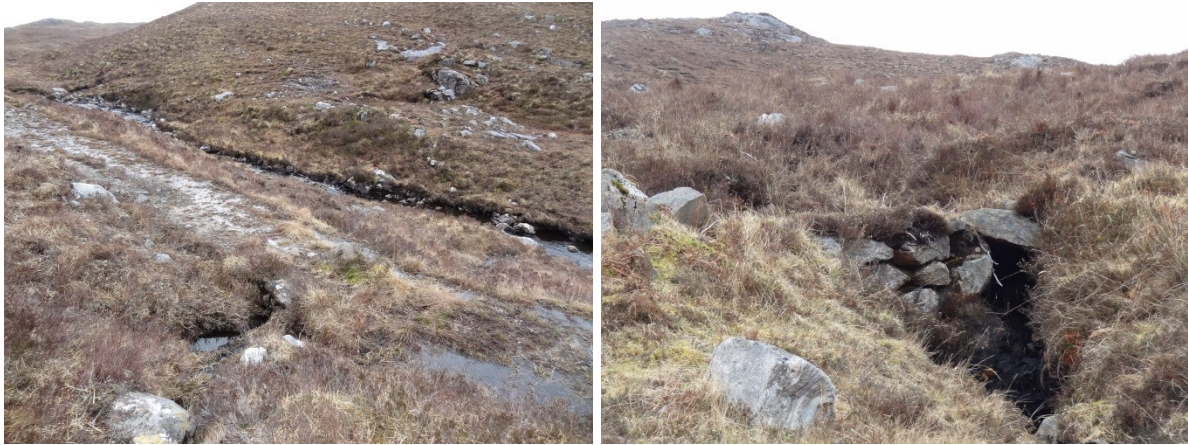
The numerous paths on Killilan Estate in Glen Elchaig were well designed and built, with SP9.04 Loch nan Ealachan displaying stone cundies (left) and a small check-dam ford.
