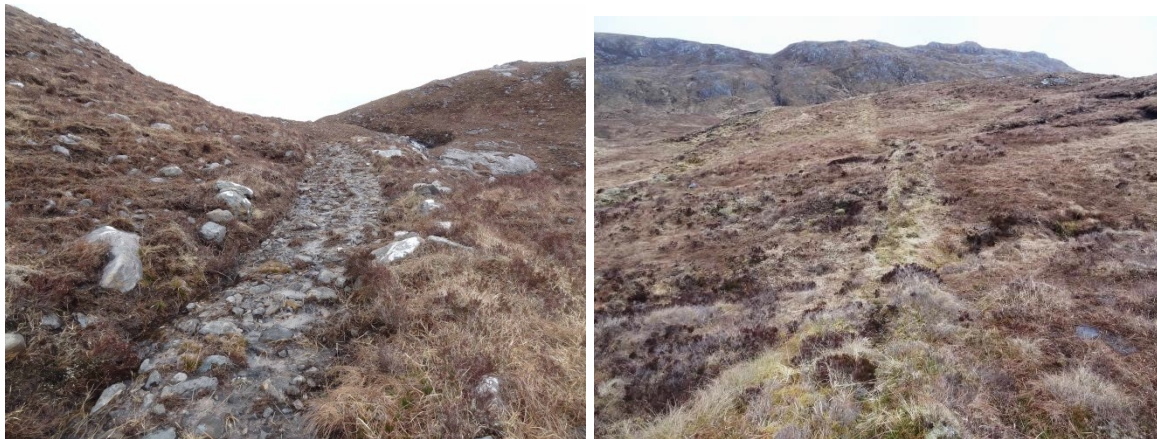
SP9.04 Loch nan Ealachan , Killilan, Glen Elchaig displays stone pitching to strengthen the scraped surface on a wet ascent, and a raised turf-bank path across a peaty moor lacking 'till' to expose or borrow.
